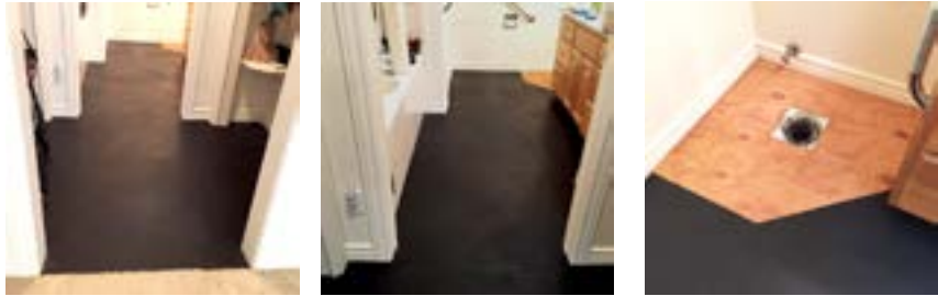
SMARTCELLS FLOORING INSTALLATION
