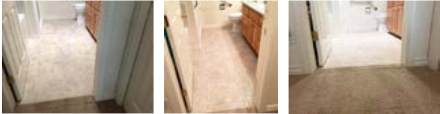
FINISHED INSTALLION WITH FLOOR COVERING
